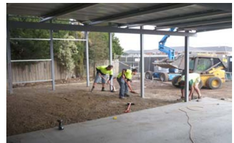
Spreading the Crush rock ready for the concrete
